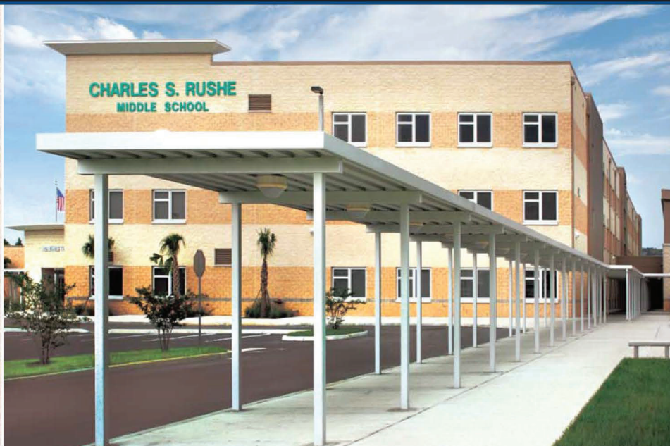
Charles S. Rushe Middle School Land O'Lakes, Florida Contractor: Skanska USA Architect: Harvard Jolly Clees Toppe Architects
